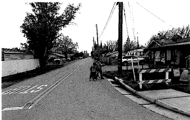
Discontinued sidewalk in Olivehurst
